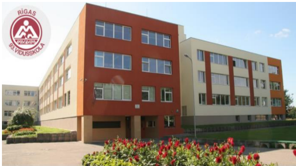
Photo 1. Building of School No. 93 in Riga - Latvia.
