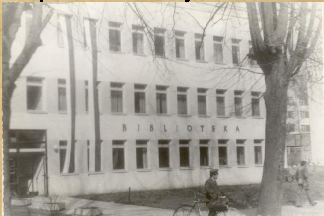
Library in the building on Mickiewicza Street
